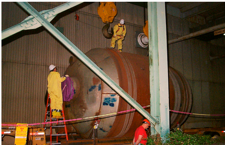
K-33 Converter Lift Complete
