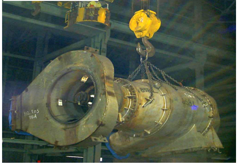
K-33 Compressor Lift
