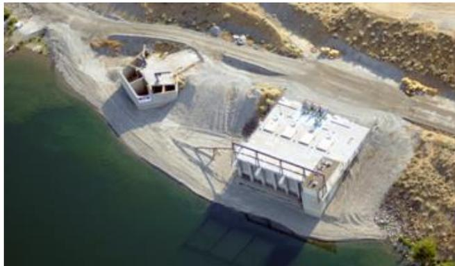
**Earthen benches used to isolate structures from the Columbia River**
