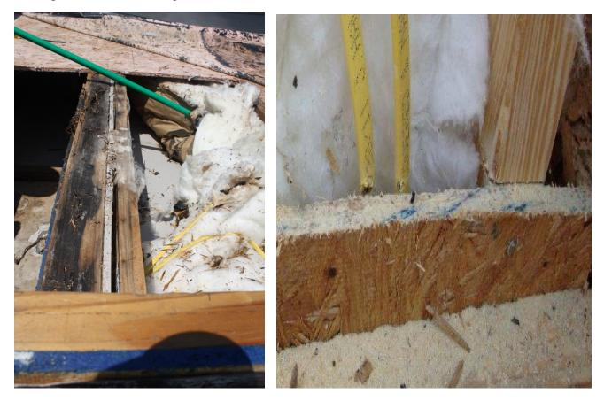
It is suspected that this circuit was installed after the walls and ceilings were in place because the wiring was not secured to the framing members. Had it been, it is likely that the cable would have been placed farther back on the stud and would not have been cut into.
