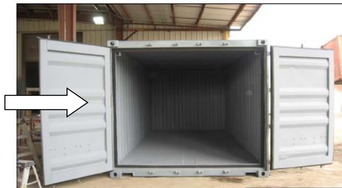
Figure L-3. Bulkhead that sandwiches between outer doors and inner seal
