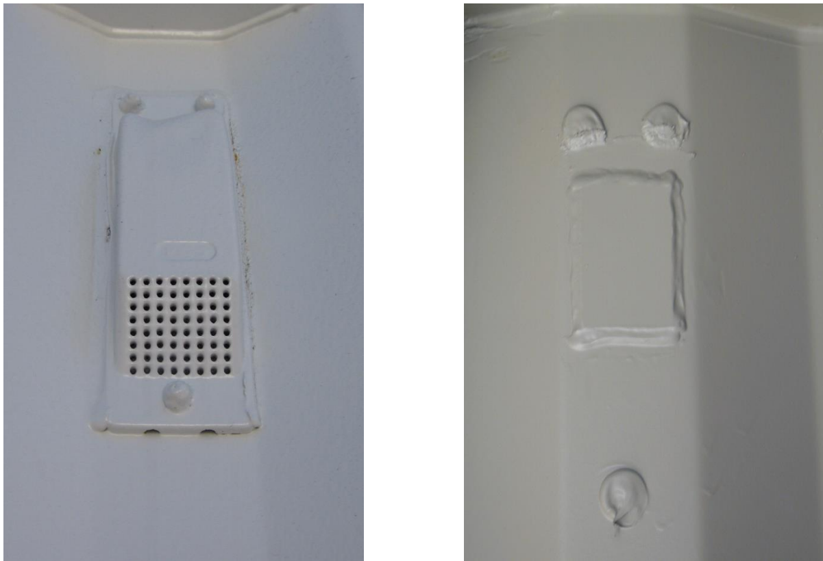
Figure L-5. Freight container vent on exterior wall (left photo). Right photo shows vent with a welded plate over the opening and sealed from the inside by welding and caulking fasteners.
