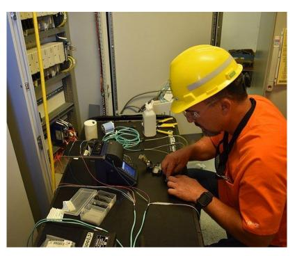
An electrician installs fiber optic cables inside an electrical powerhouse for the Effluent Management Facility at the Hanford Site's Waste Treatment and Immobilization Plant.
