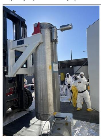
During a planned maintenance outage, workers change out spent 27,000-pound filter columns in the Tank-Side Cesium Removal System and place them on a nearby storage pad.
