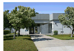
Figure 1. The LLNL Heavy Element Facility
