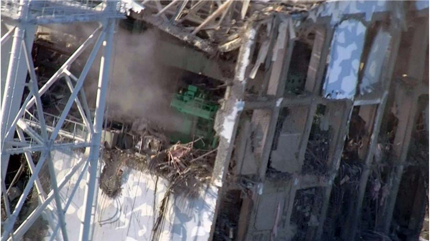
March 17, 2011 Tepco image of damage to Unit 4.
