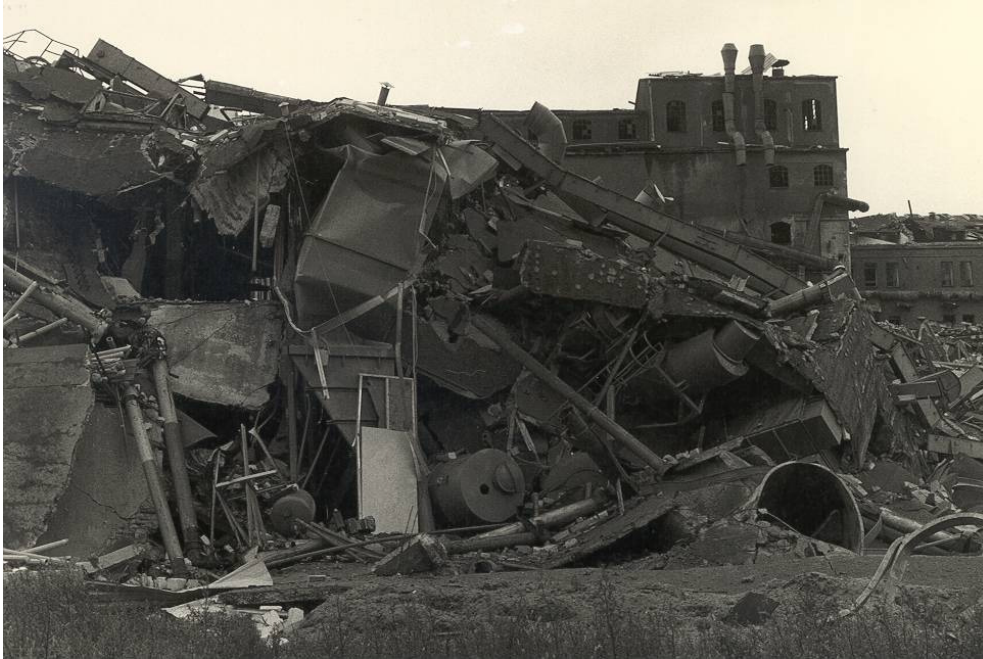
Figure 21.1 Remains of an oil seed plant after a UVCE, Copenhagen 1982
