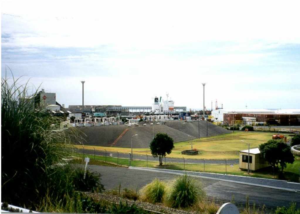
Figure 8.6 Mounded vessel storage for LPG
