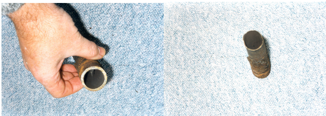
Figure 7.9 Two ends of a pipe section corroded under lagging when water soaked in.
