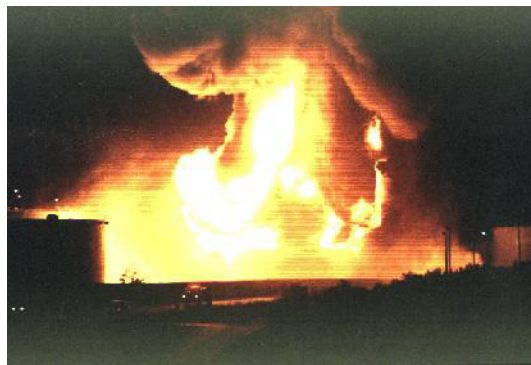
Figure 10.2 Floating roof tank boilover
