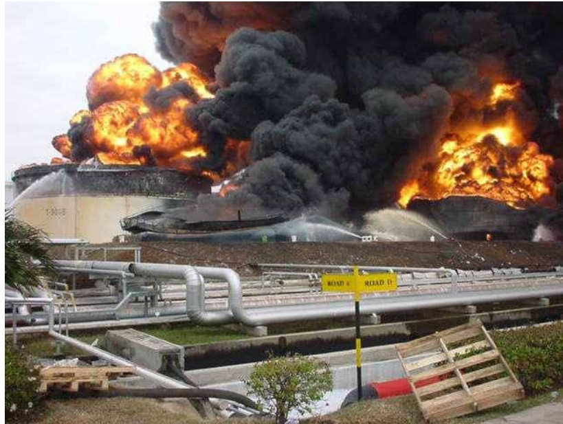
Figure 10.5 Domino effects from floating roof tank fire
