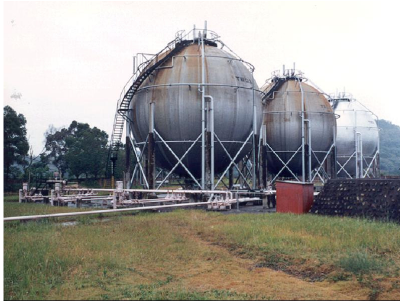
Figure 8.3 LPG spheres
