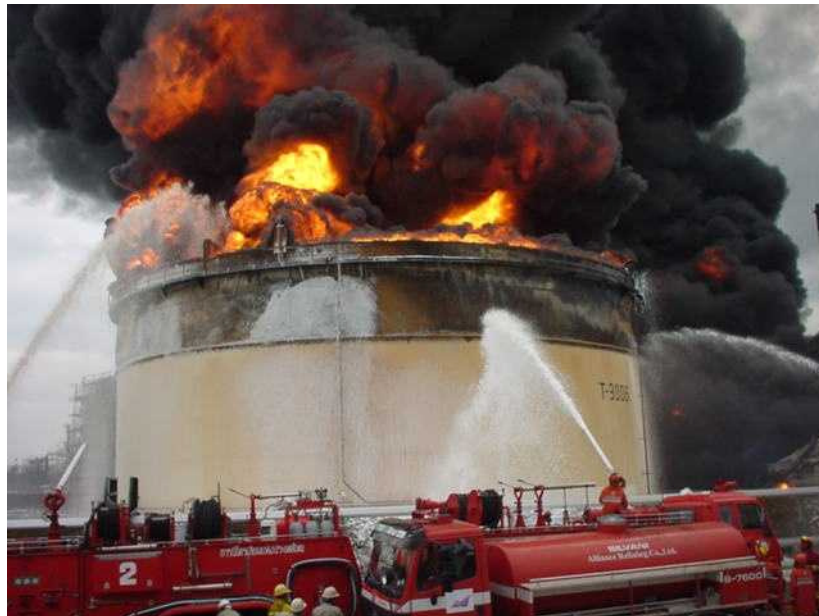
Figure 10.4 A floating roof tank fire
