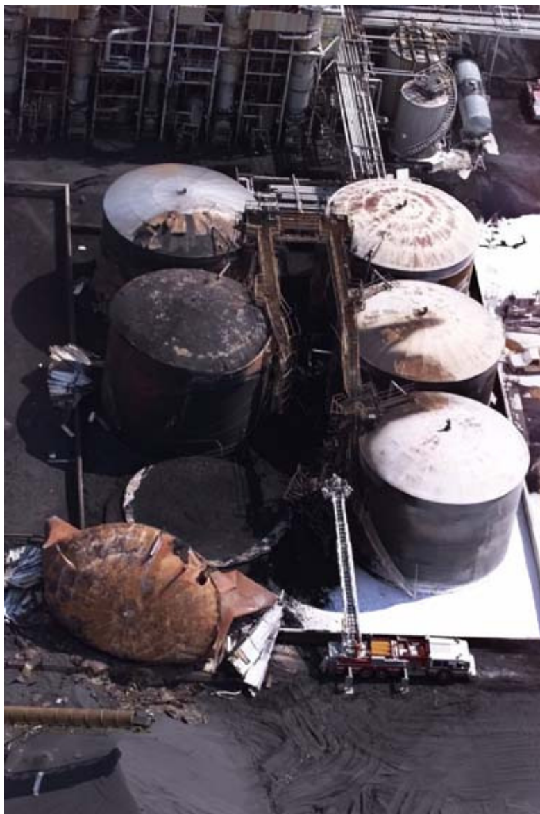
Figure 9.2 Sulphuric acid tank explosion/collapse at Motiva
