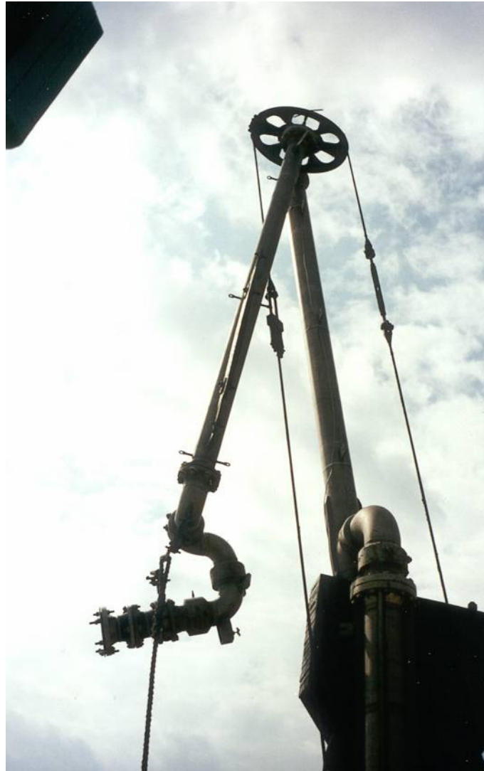
Figure 11.1 A loading arm for coupling ship to shore terminal piping.
