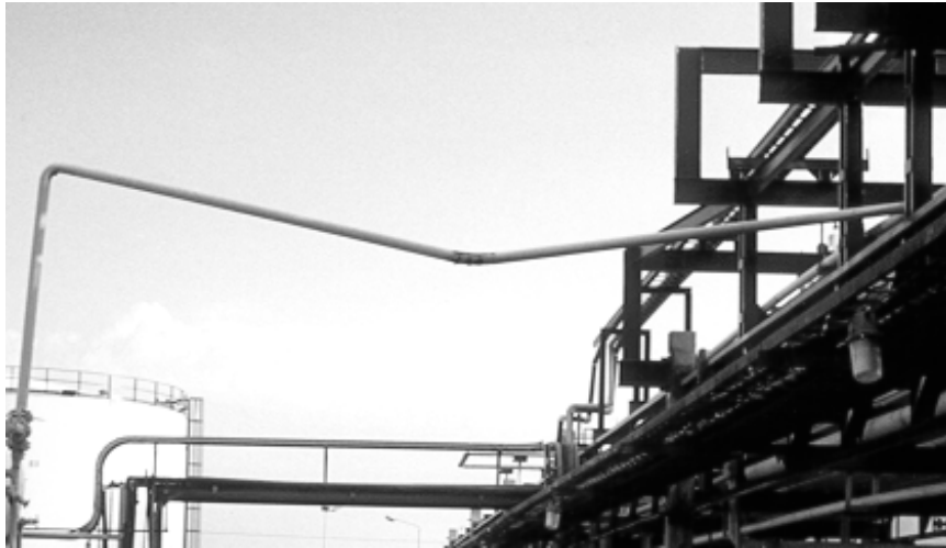
Figure 7.7 Overhead pipe, hit by crane and leaking
