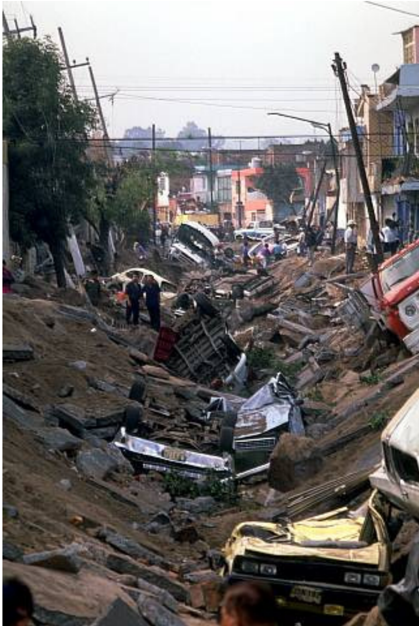
Figure 21.2 Debris after a gasoline vapour explosion in a sewer, Guadalajara, 1994
