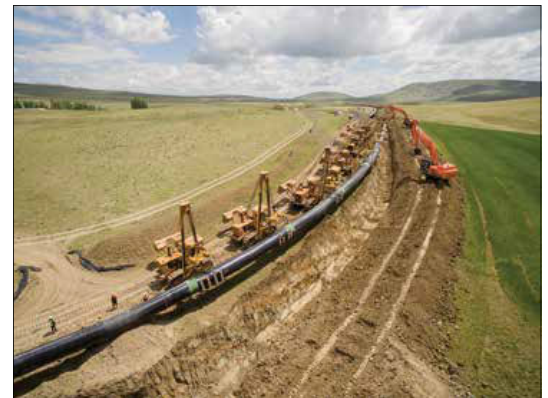
Pipeline installation (Photo courtesy of TANAP Natural Gas Transmission Co.)
