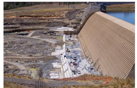
Above and below: Paradise Dam was the first roller compacted dam built in Australia. Images courtesy of Rod Savidge.
