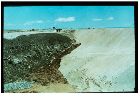
A leak forms in the Teton Dam as the dam is put into service, June 5, 1976
