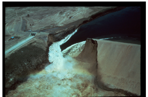
Fully breached, water pours through the opening caused by the leak.
