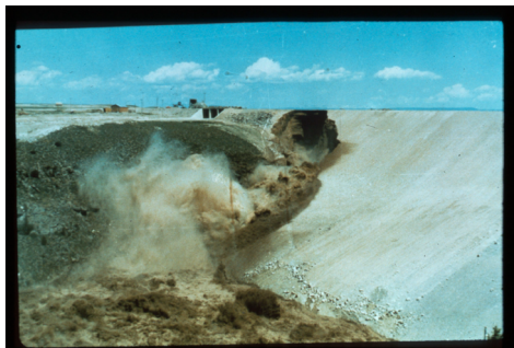
The dam begins to give way under the immense water pressure behind it.
