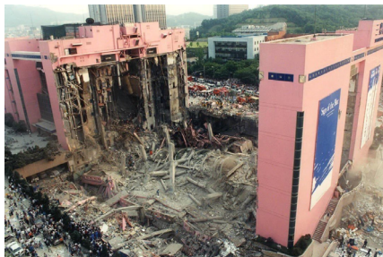
The entire middle section of the building collapsed when the AC units fell through the roof.
