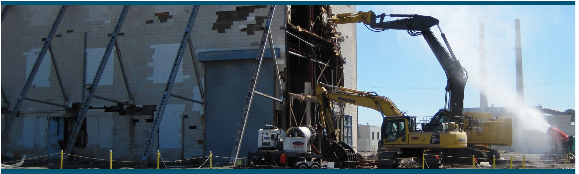
Demolition at Hanford Site
