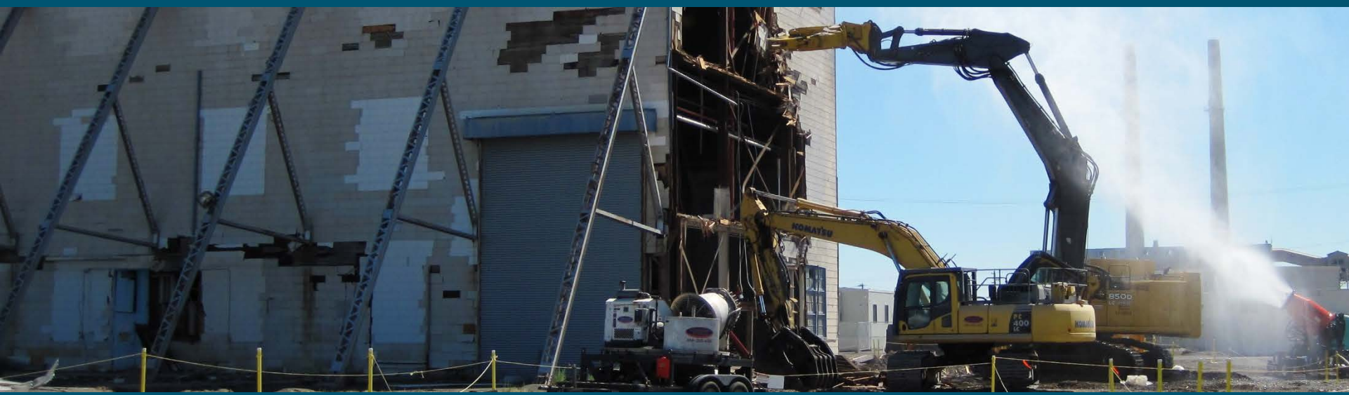
Demolition at Hanford Site
