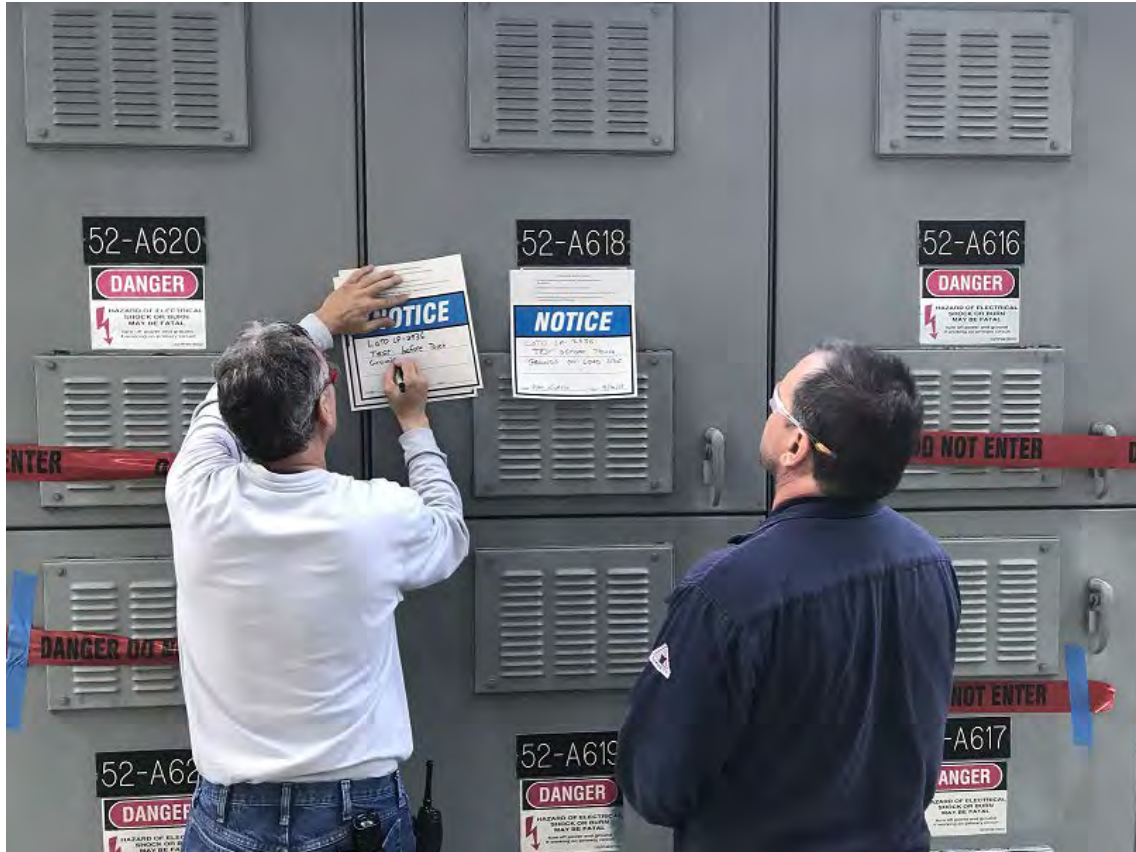
Figure 7B – Signage Installation on back of substation cubicles
