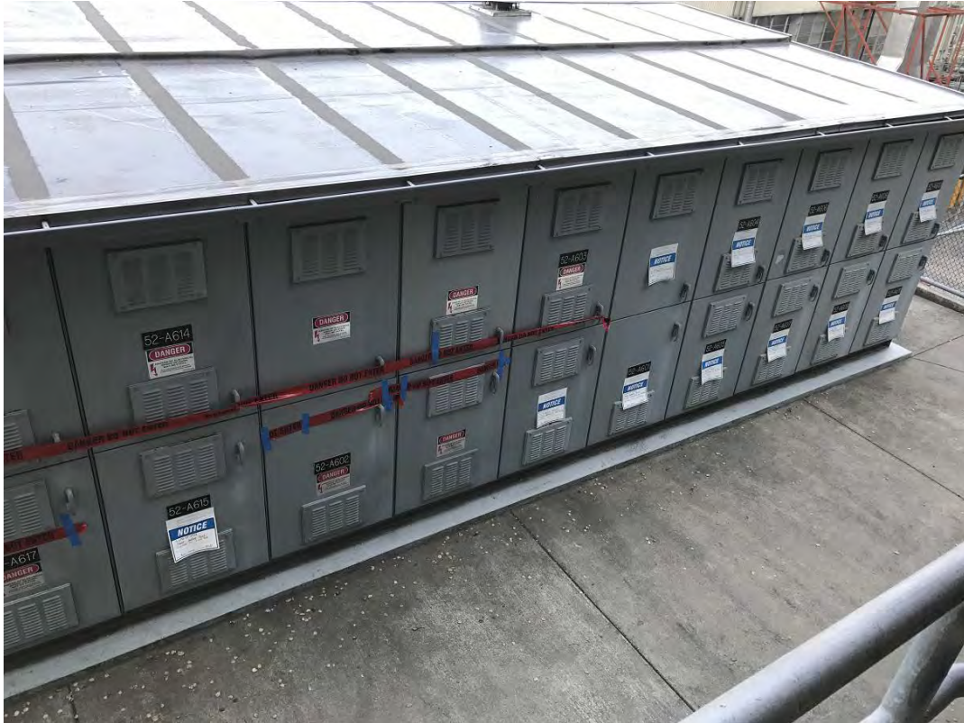
Figure 7D – Substation view once all signs and barricade tape installed
