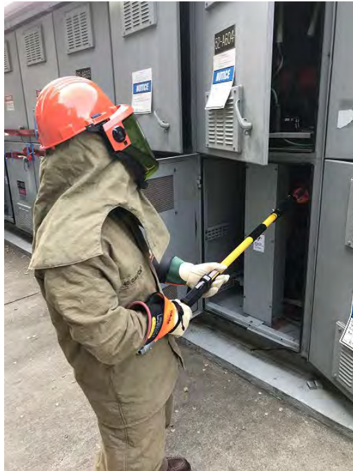
Figure 8A – Magnetic Signs used on energized cubicles
