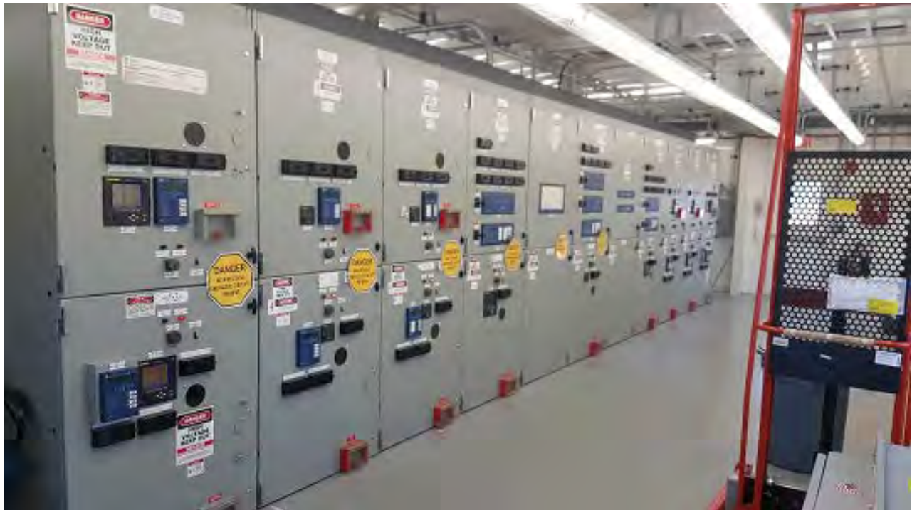
Figure 8B – Magnetic Signs Installed (front view)
