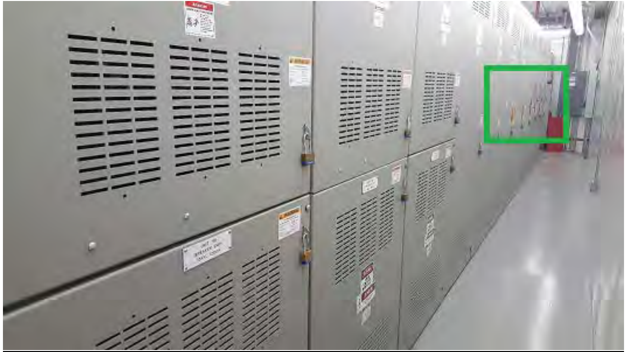
Figure 8D – Magnetic Signs Installed (vertical opening)
