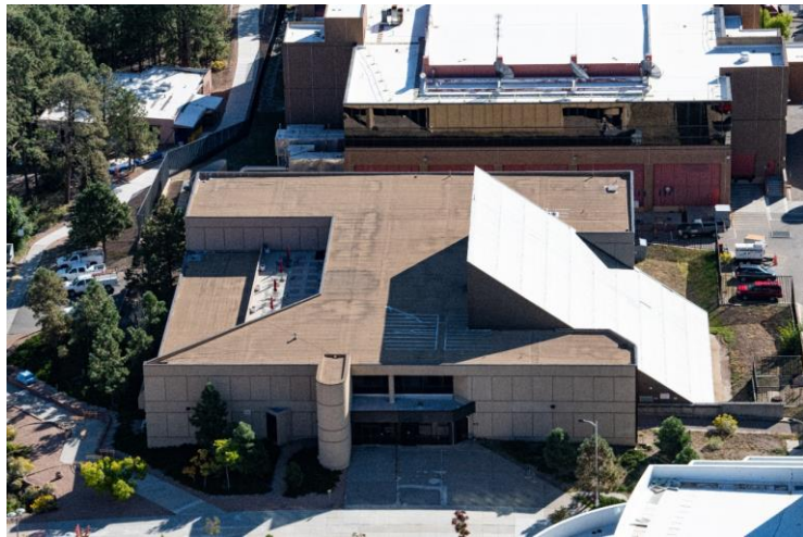
Research Library built with slanted roof for solar panels, as was the Otowi Building.
