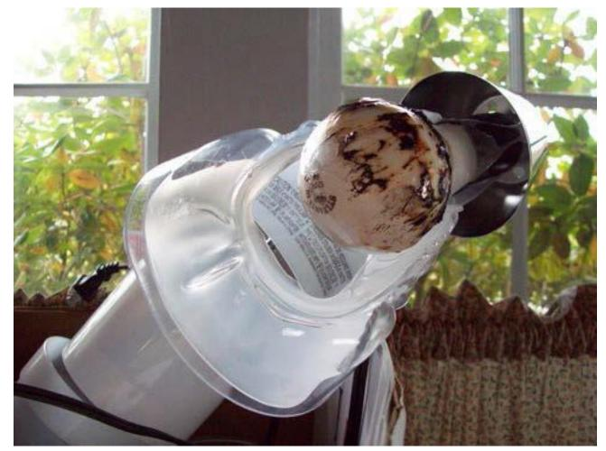
The bulb was plenty bright (100 watts), but that is (was) a 40-watt fixture.
