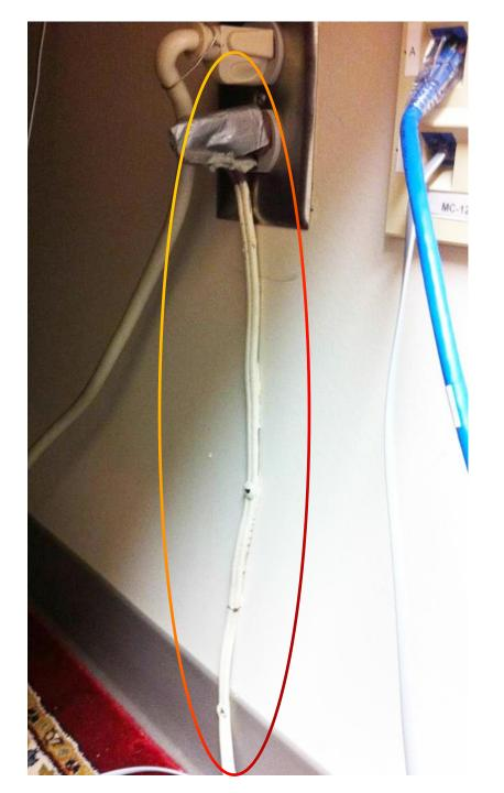
This cord had been stapled and tacked to the wall, for some reason. The cord ran under a carpet to a coffee pot and radio. The duct tape is just the final, unsurprising detail. The perfect finishing touch!
