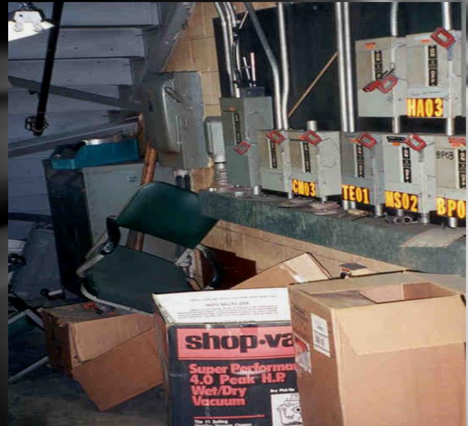
Poor access to disconnects.
