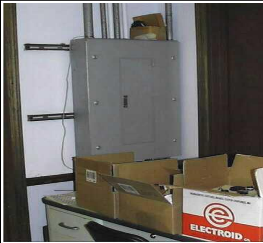
Blocked access to circuit breaker box.
