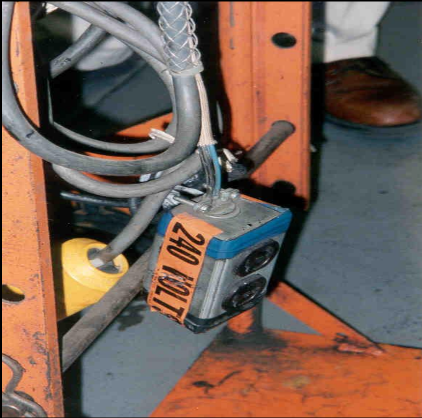
Improper and damaged extension cord.
