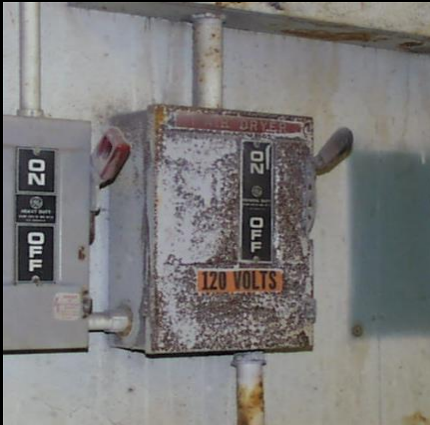
Acid corroded electrical disconnect.
