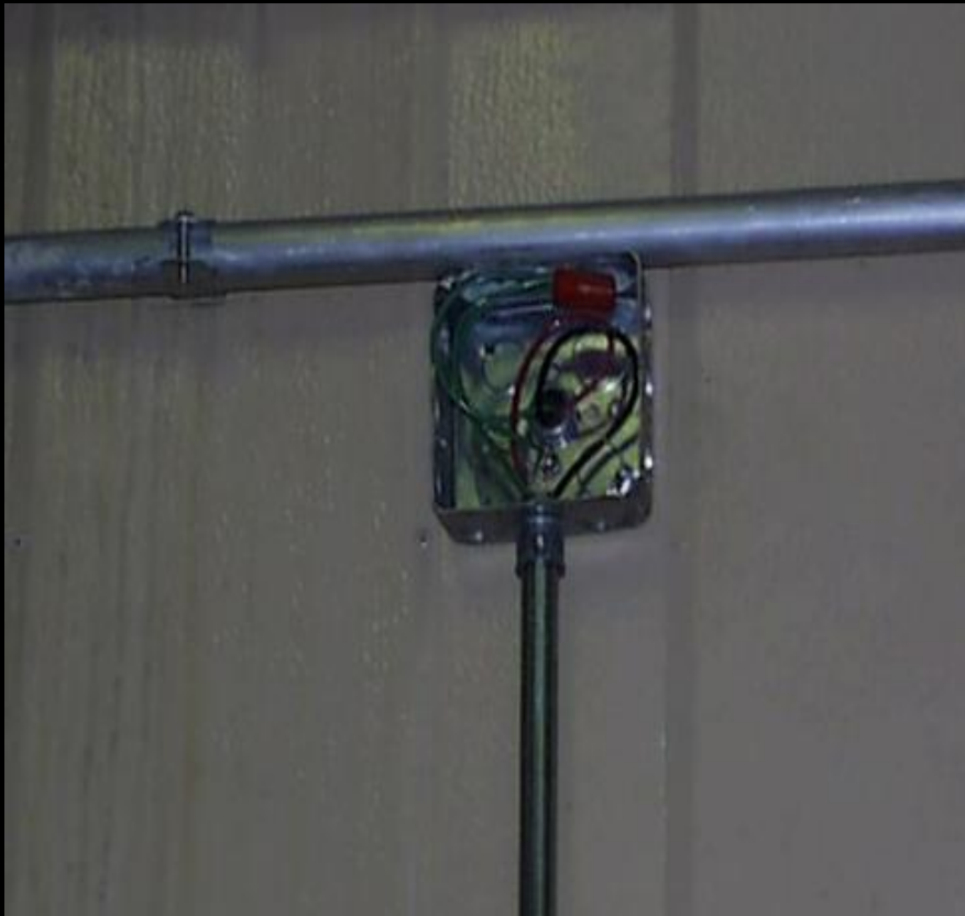
Missing cover on junction box.
