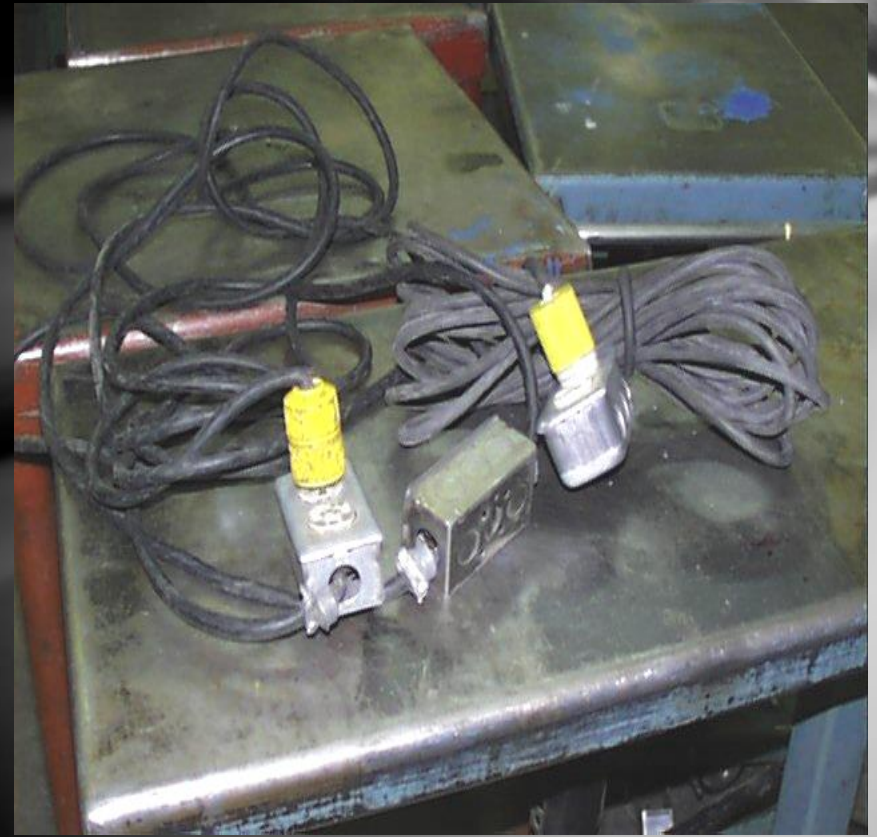
Improper and damaged extension cords.
