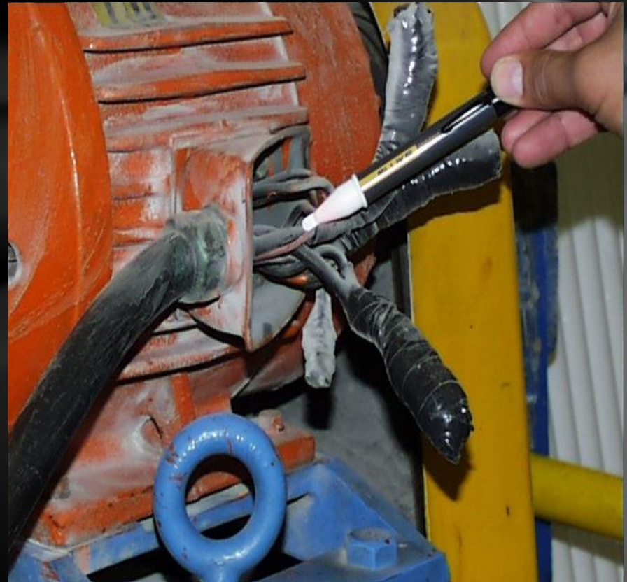
Exposed wiring into motor housing.
