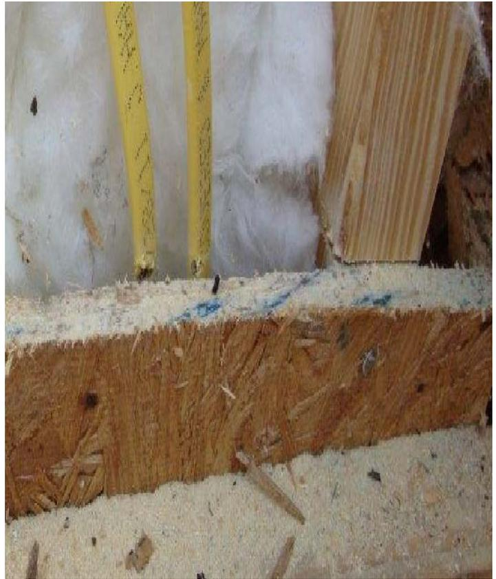
It is suspected that this circuit was installed after the walls and ceilings were in place because the wiring was not secured to the framing members. Had it been, it is likely that the cable would have been placed farther back on the stud and would not have been cut into.
