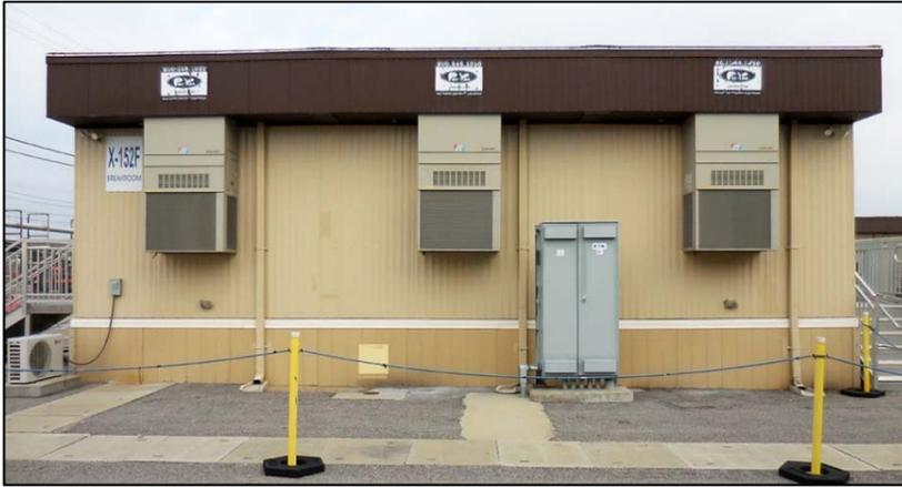
Additionally, 550.32(F) specifies the mobile home disconnecting means must be installed so the bottom of the enclosure containing the disconnecting means is not less than 600 mm (2 ft.) above finish grade or the working platform. The disconnecting means must be installed so that the center of the grip of the operating handle, when in the highest position, is not more than 2.0 m (6 ft. 7 in.) above the finished grade or working platform.
