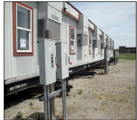
Section 550.32(A) also permits the service equipment to be located remote from mobile home provided a disconnecting means that is suitable for use as service equipment is located in sight from and not more than 9.0 m (30 ft.) from the exterior wall of the mobile home it serves. In the photo to the right, the service equipment is located at the far end between the two poles.
