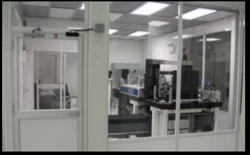
By walls and filtered windows (Room)
