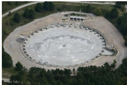
Cooling Tower (aerial, at completion)
