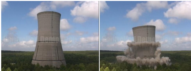
Cooling Tower (before)
