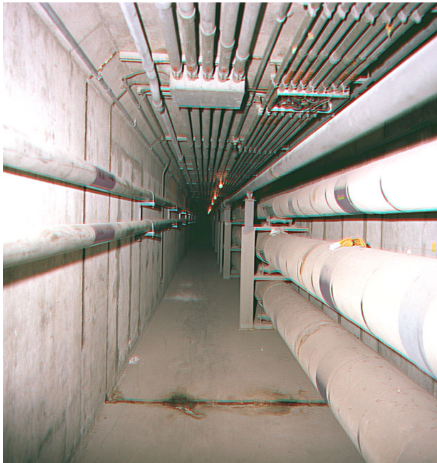
Figure 18. Interior of the GEEL tunnel looking toward the northeast
