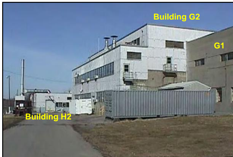
Figure 2. SPRU Facilities Before the Start of the Current Decommissioning Project, Looking North (from ERG 2006a)
